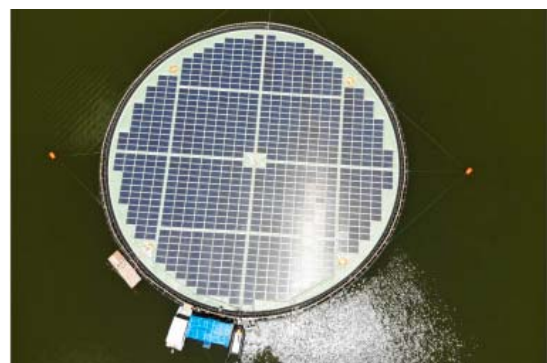
Figure 39 Large-scale polymer offshore floating structure for photovoltaics (Xu et al., 2022)
