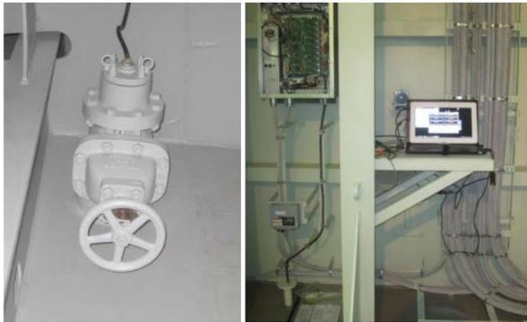
Figure 8: MLDS equipped on 14,000TEU container ship (Left: the gate valve for the transducer of the MLDS at the bottom, Right: the transceiver of the MLDS and PC for analysis in the steering gear room) (Inukai 2019)
